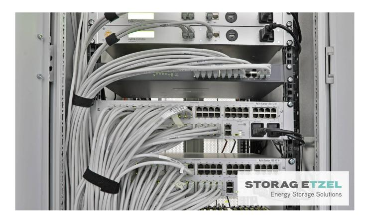
Redundancy for maximum safety on the site of STORAG ETZEL's cavern storage facility in Friedeburg, Lower Saxony. The lower two components are the MultiCenter for control room operation with MultiConsoling® – here in double version for maximum safety.
