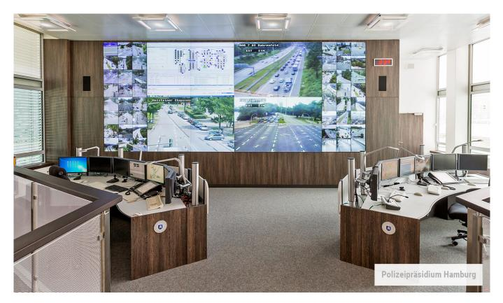
A visual and technical asset for traffic monitoring: the <u>Hamburg traffic control center</u>. Triggering height control in the Elbe tunnel, collisions on the main arterial roads or traffic jams – the employees can switch on the required camera images from any location in the event of an alarm. The advanced video wall technology enables the police to undertake virtual "patrols" on the video wall.
