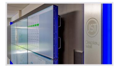
JST large display technology: JST pays particular attention to the details. This can be seen, for example, in the design of the <u>large display wall</u> with high-quality brushed stainless steel design strips, accentuating AmbientLight and flush-fitting loudspeaker systems. The AmbientLight can, for example, flash red in the event of a critical alarm – in other words, it is "event-controlled".
