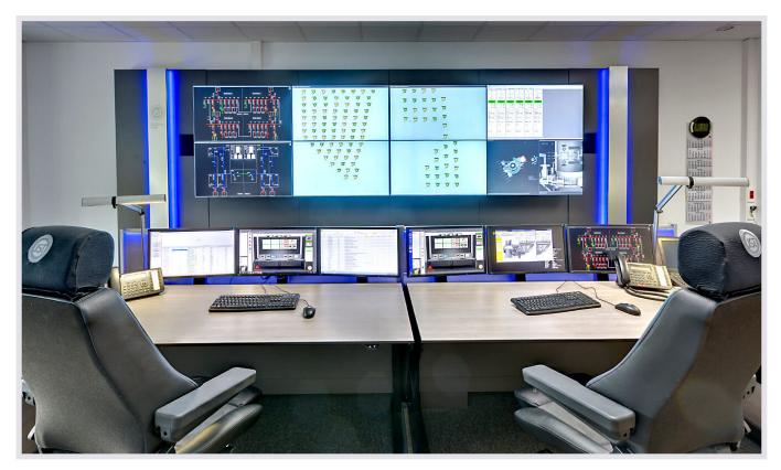
JST control center concept: In the Bremerhaven Adwen <u>control center</u>, operators benefit from the extensive wealth of experience of the JST specialists. Workstations that meet the latest technical and <u>ergonomic</u> requirements, as well as a carefully thought-out <u>room concept</u> and proactive visualisation of the various systems characterise the control room.
