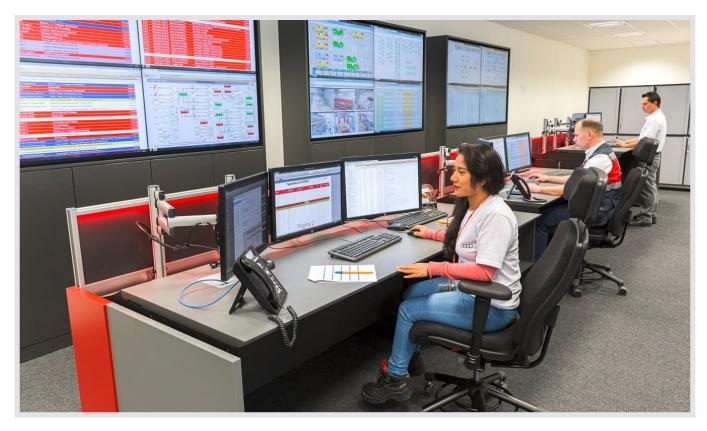
© AUDI AG | JST control room workstation: A total of <u>35 operator workstations</u>, designed on the basis of current occupational health recommendations for work in control rooms, were installed by JST in the Audi <u>production control room</u> in San José Chiapa, Mexico. <u>Ergonomic aspects</u> played just as much a role as a special demand for <u>high availability technical solutions</u>.
