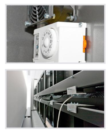
A switching unit makes it possible to regulate the ventilation individually via thermostat.
