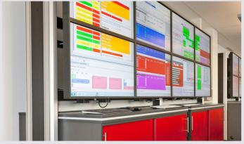
JST large display walls: A total of 16 high-end displays for 24/7 continuous operation, distributed over two units, were installed in the Frankfurt control center. Business displays integrated in the JST display rack with media boards – the racks are equipped with roller runners for the case of revision.
