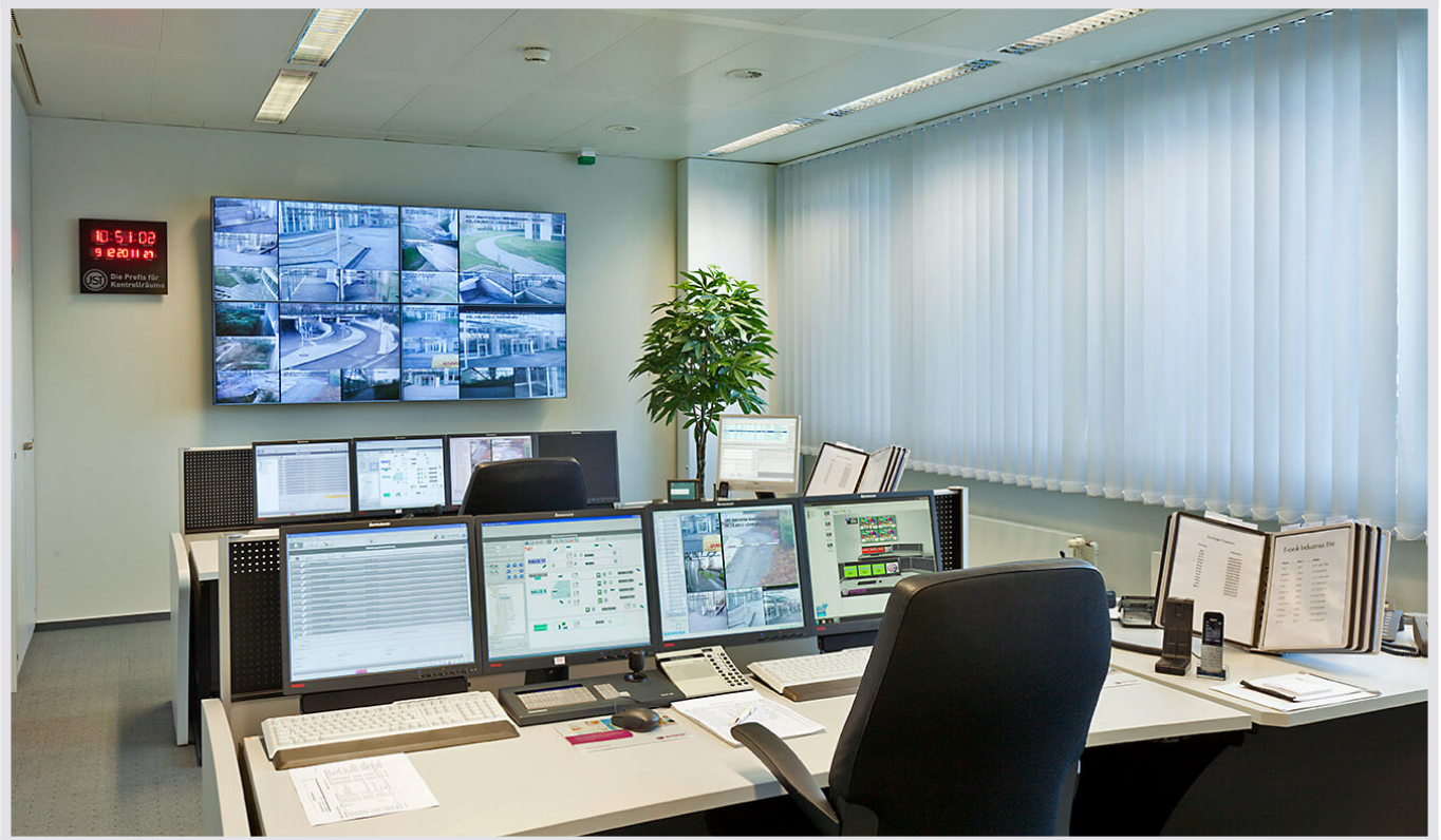
Evonik Essen: Safety headquarters
