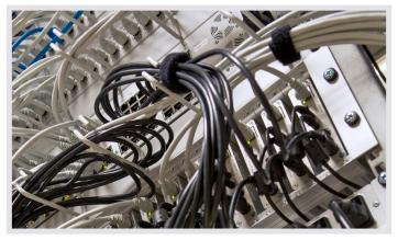
**JST MultiConsoling**\*: View of the technology for the myGUI user interface – the MultiCenter is located in the upper part of the picture, below the grabbers to which the individual computers are connected and thus connected to the MultiCenter.
