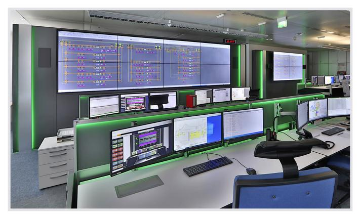
JST control room: Green <u>AlarmLight at workstations</u> and <u>large screen wall</u> - a signal for trouble-free system operation. If the <u>PixelDetection</u>® software detects deviations, the operators in the <u>control room of Charité CFM Facility Management GmbH</u> are alerted by flashing red light and acoustic signals.
