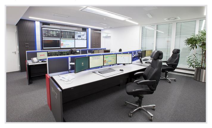
JST control room concept: With the new <u>integrated control center</u>, Stadtwerke Gießen was able to combine its two previous power supply control centers. Workstations that meet the latest <u>technical</u> and <u>ergonomic</u> requirements, as well as a carefully thought-out room concept and <u>proactive visualisation</u> of the various systems characterise the control room.
