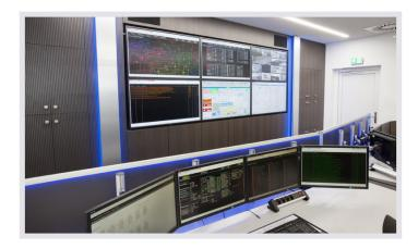
JST DisplayWall®: Perfect in design and workmanship – the <u>DisplayWall</u>®. Design strips with high-quality aluminium brushed surfaces and the AlarmLight give the monitor wall a special look. The 46 inch <u>LCD displays</u> were perfectly fitted into the <u>sound-absorbing covering of the large display screen</u>.
