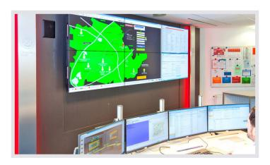
JST <u>large display wall</u>: The JST<u>DisplayWall</u> keeps the entire control center team informed about the most important events in real time. The <u>JST-PixelDetection</u>® software ensures automatic source switching to the DisplayWall. At the same time the coloured AlarmLight ensures that no alarm is lost.
