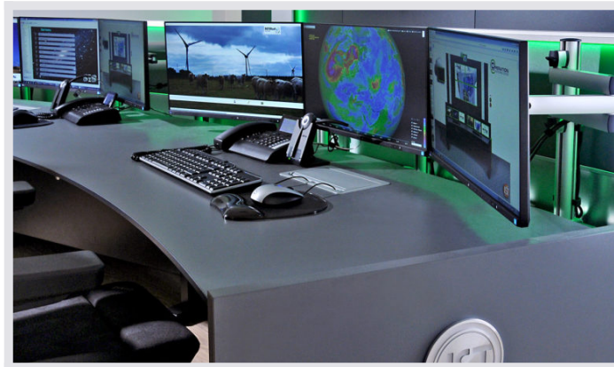
JST-Operator desk: With a clear number of monitors and taking into account all ergonomic aspects, the perfect workplace for control center staff: side view of the Stratos operator console.
